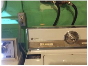
The hookups for the dryer are properly installed and in serviceable condition. The dryer itself was operated through a partial cycle, however we did not confirm the complete operation of the cycle timer.
