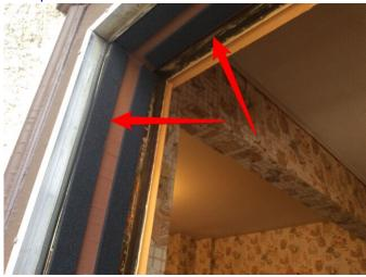
The upstairs exterior door is deteriorated. We recommend it be repaired or replaced.
