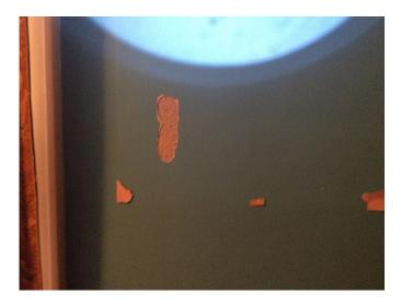
Front porch ceiling and wall show signs of past water damage. I suspect damage was caused by ice dams. Roof should be monitored for ice buildup and snow removed when possible.
